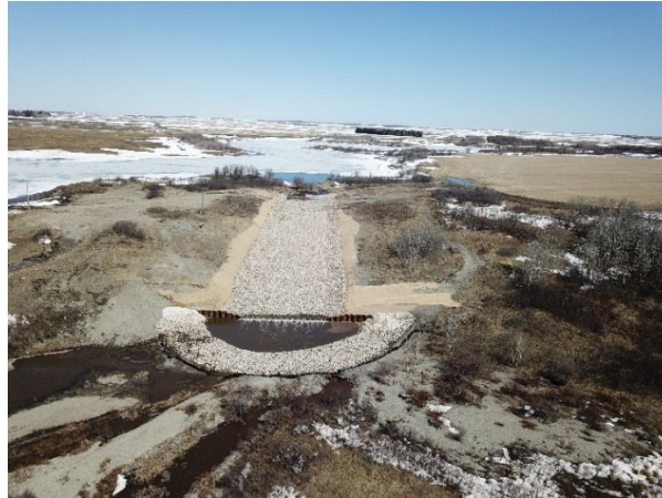
completed riprap lined auxiliary spillway (Spring 2023)
