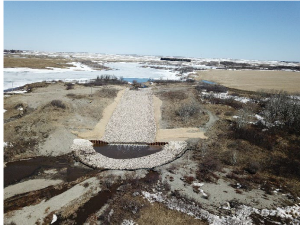
completed riprap lined auxiliary spillway (Spring 2023)
